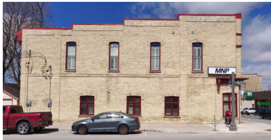
191 Main Street (Hwy 6) Side
