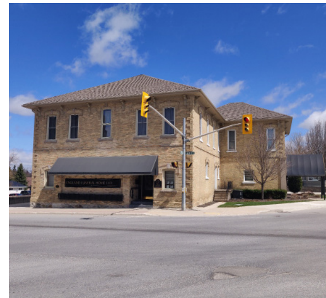
294 Main Street (Hwy 6) - side
