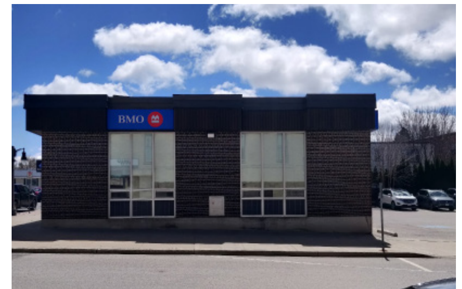
201 Main Street (Hwy 6) Side
