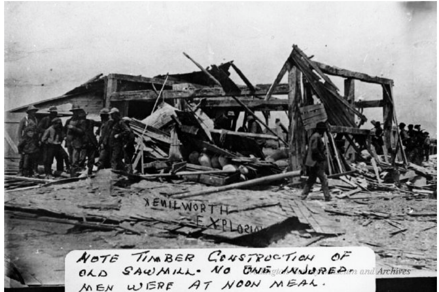
The remains of the Kenilworth Mill following its explosion on May 19, 1910. (Photo from Wellington County Museum and Archives)
