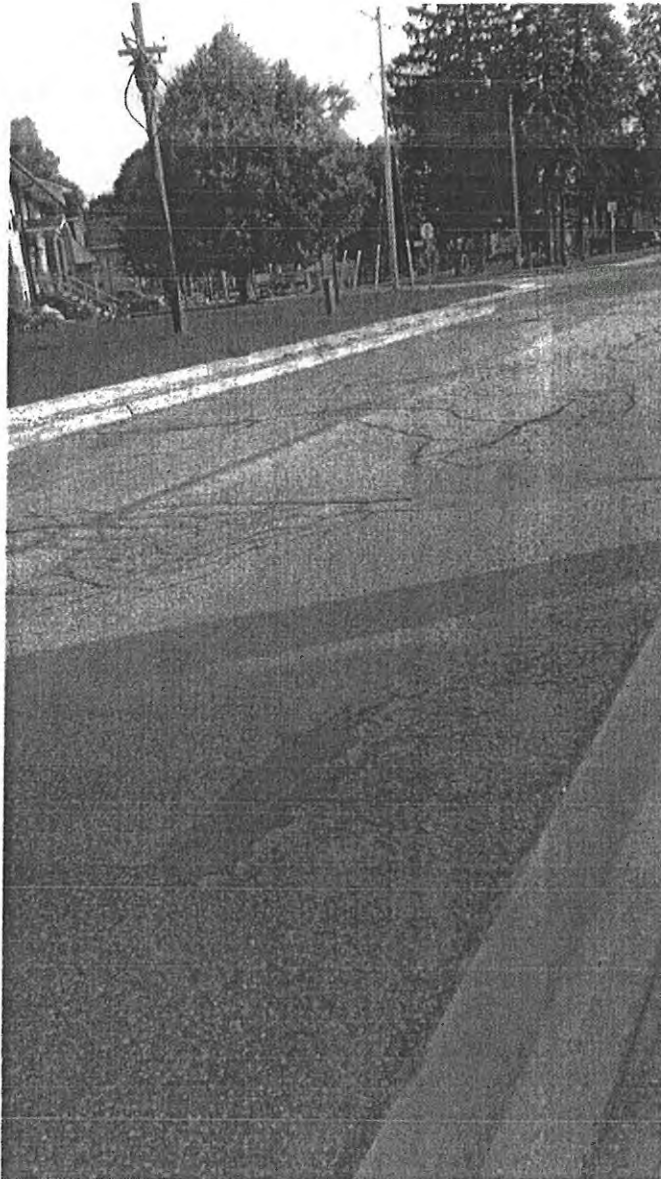
Looking east from south side of road, west of William Street.
