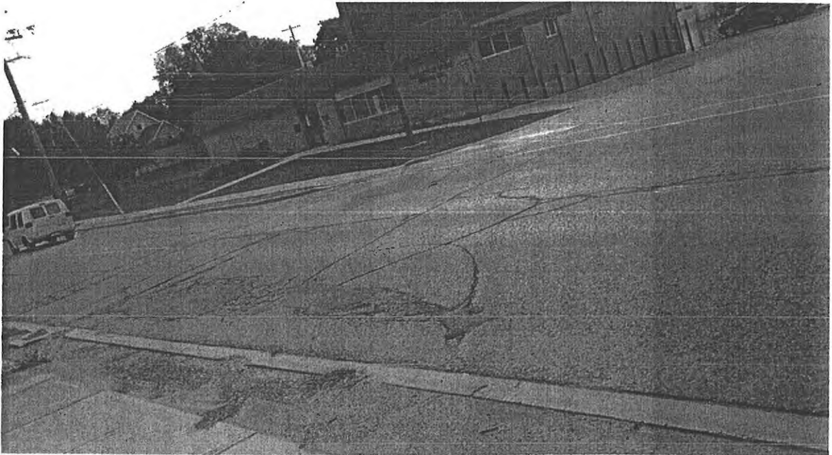
Looking south from north side of road at Arthur Street intersection.
