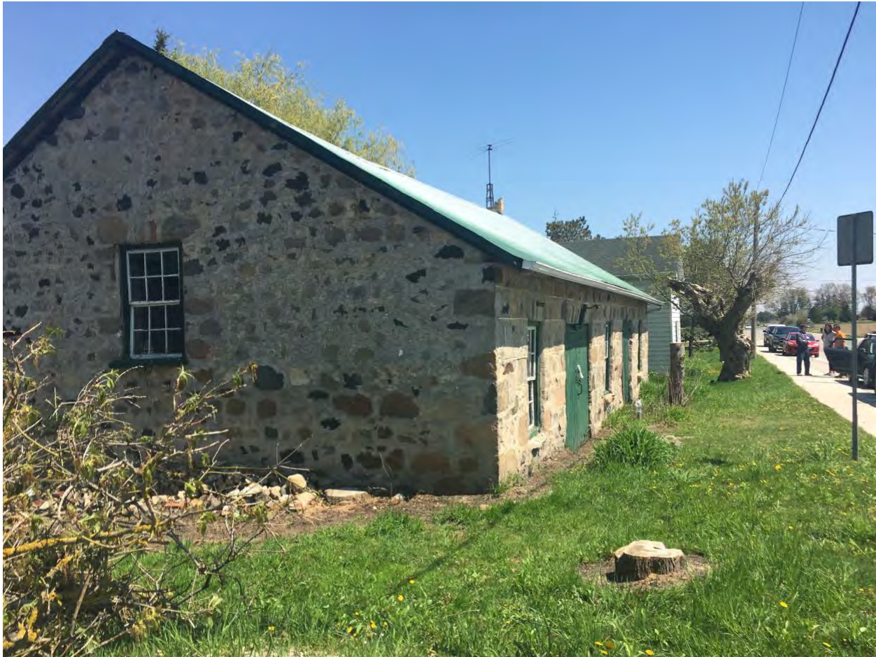
View of front of the Blacksmith Shop looking south along Hwy 6.
