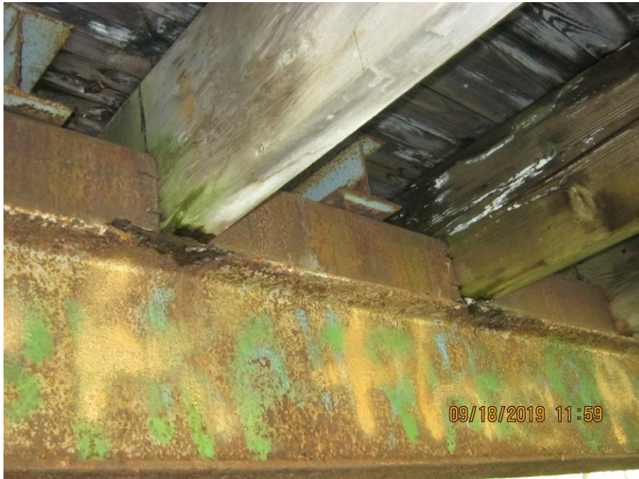
Cross beam - top flange damage
