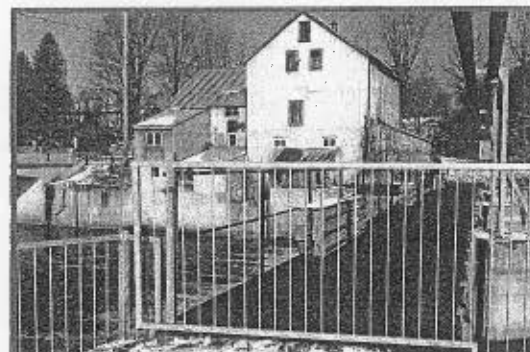
New gate and railings installed at Pioneer Conservation Area.
