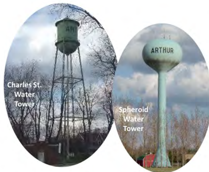
Figure 4-31: Water Towers serving the Arthur Community
