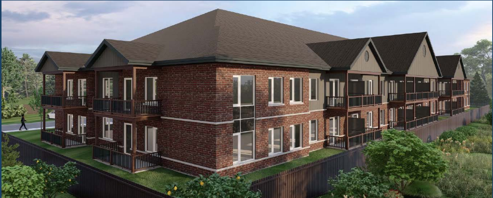
View of front building, looking north-west
