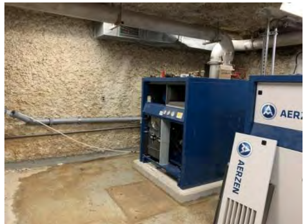
WWTP Work Site: Week 51- Photo 12.
