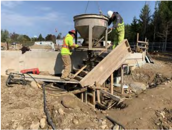
WWTP Work Site: Week 51- Photo 3.
