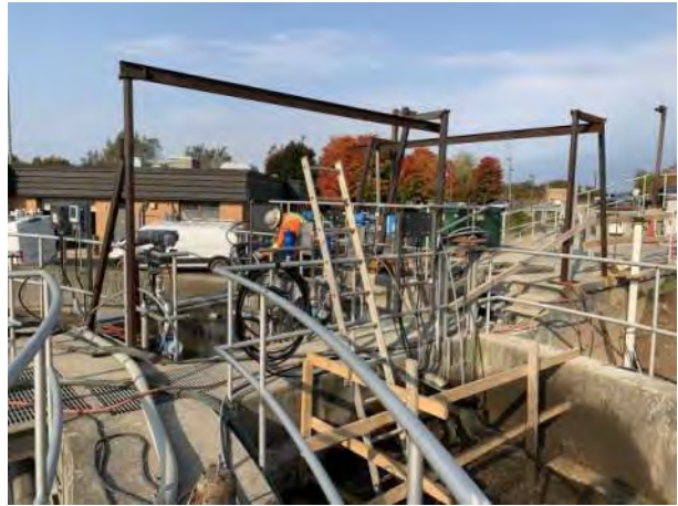
WWTP Work Site: Week 51– Photo 14.
