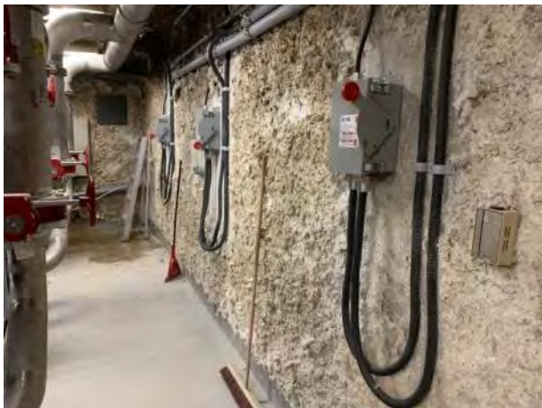
WWTP Work Site: Week 51- Photo 11.
