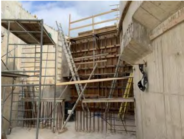
WWTP Work Site: Week 50- Photo 1.
