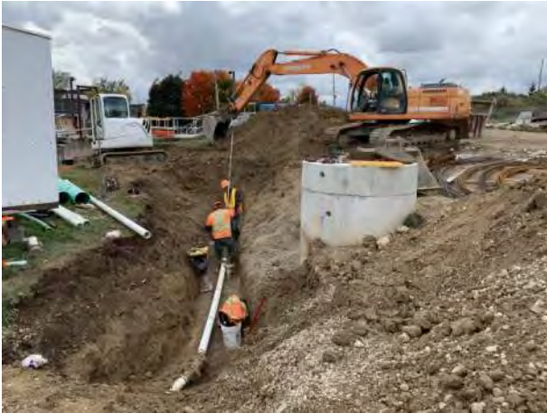
WWTP Work Site: Week 50- Photo 9.
