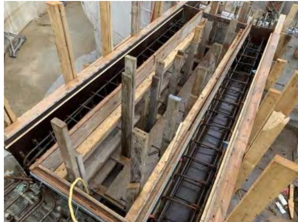
WWTP Work Site: Week 50 - Photo 2.
