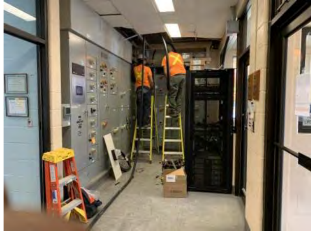
WWTP Work Site: Week 51- Photo 8.
