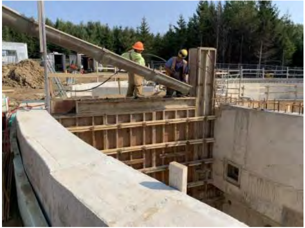
WWTP Work Site: Week 51 - Photo 2.
