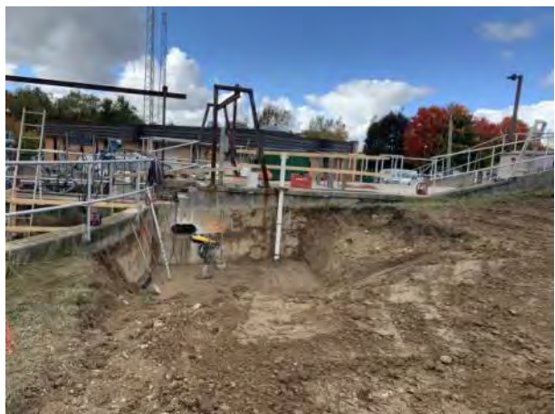
WWTP Work Site: Week 50- Photo 10.
