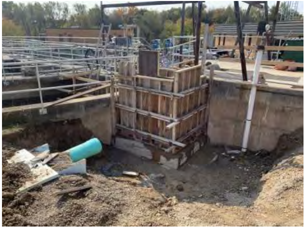
WWTP Work Site: Week 51- Photo 4.
