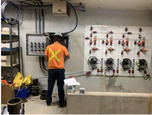
SAN PS Work Site: Week 51- Photo 7.
