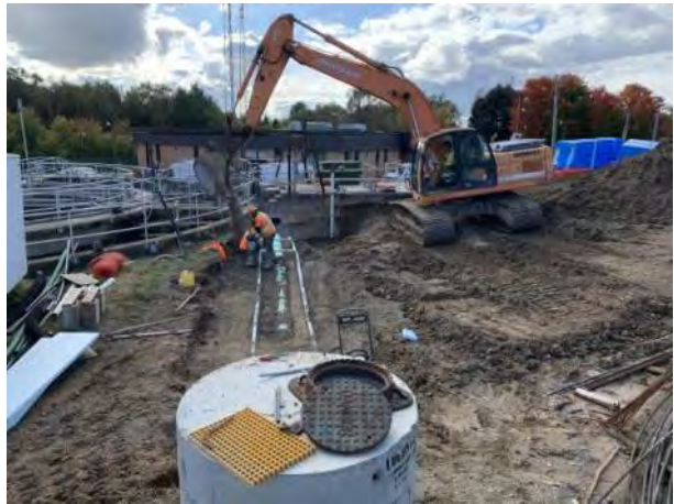
WWTP Work Site: Week 50- Photo 8.
