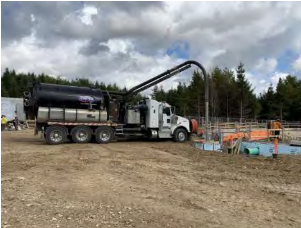
WWTP Work Site: Week 50- Photo 3.
