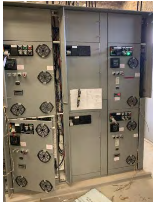
WWTP Work Site: Week 50- Photo 14.
