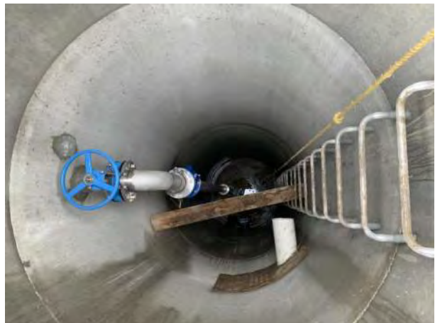
WWTP Work Site: Week 50- Photo 4.
