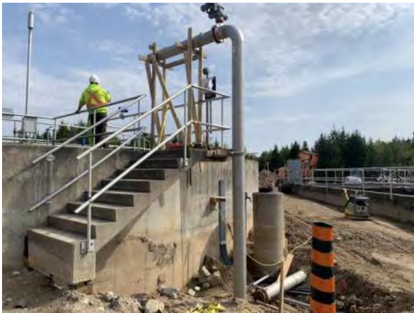
WWTP Work Site: Week 51- Photo 5.
