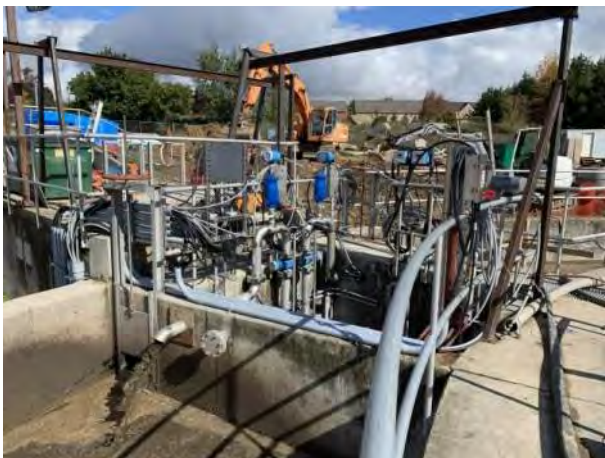
WWTP Work Site: Week 50- Photo 5.
