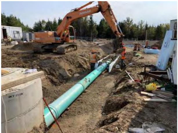
WWTP Work Site: Week 51- Photo 6.
