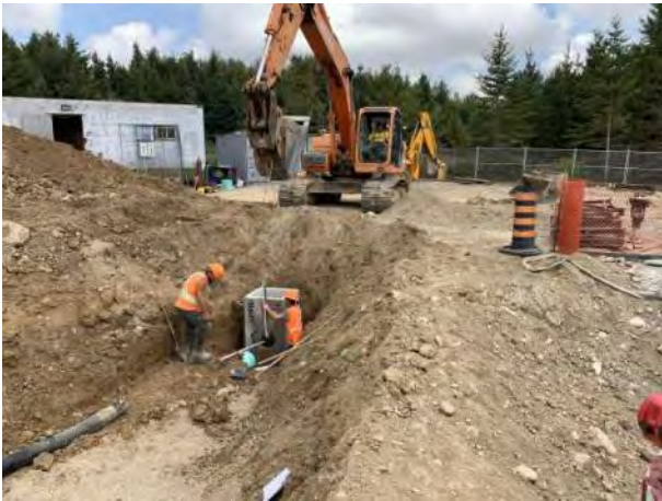
SAN PS Work Site: Week 50- Photo 7.
