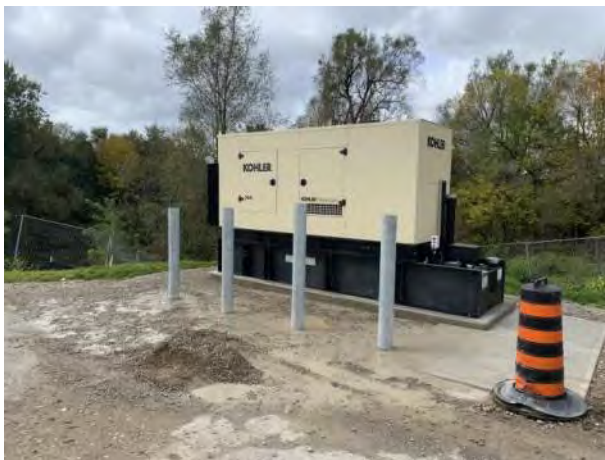
WWTP Work Site: Week 50- Photo 15.
