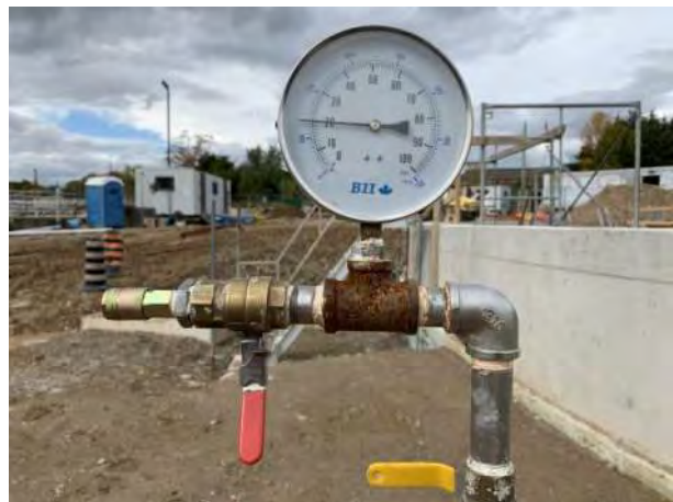
WWTP Work Site: Week 50- Photo 6.
