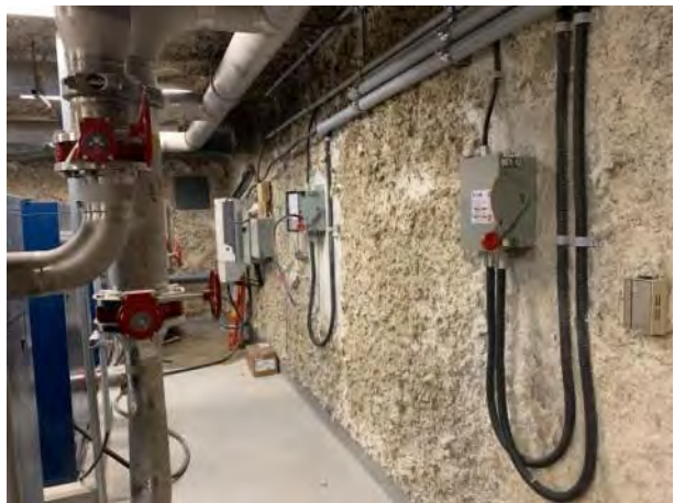
WWTP Work Site: Week 50- Photo 12.
