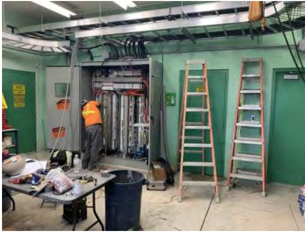
WWTP Work Site: Week 50- Photo 13.
