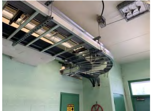
WWTP Work Site: Week 51- Photo 10.
