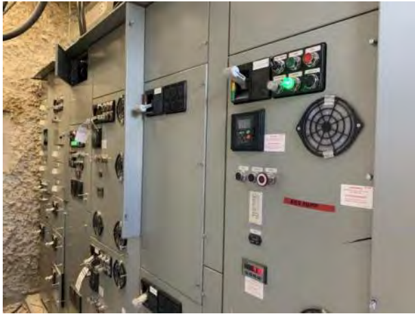
WWTP Work Site: Week 51– Photo 13.
