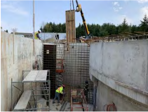
WWTP Work Site: Week 51- Photo 1.
