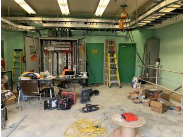
WWTP Work Site: Week 51- Photo 9.
