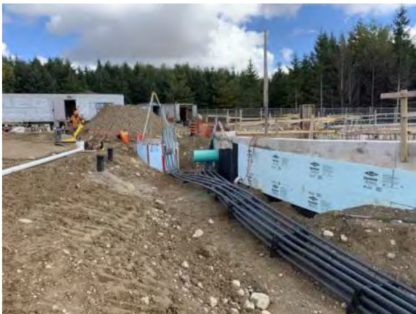
WWTP Work Site: Week 50- Photo 11.
