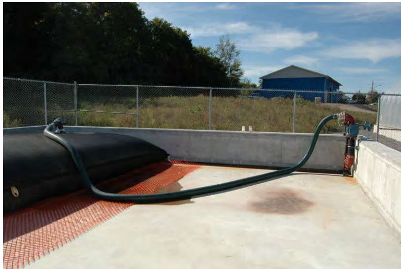
Geotube® Dewatering Cell Constructed of concrete
