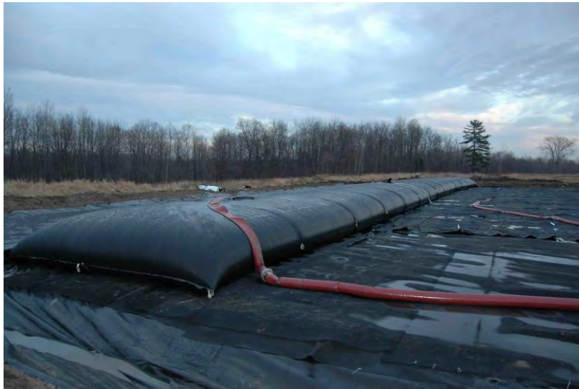
Geotube® Dewatering Cell Constructed using geo-membrane liner
